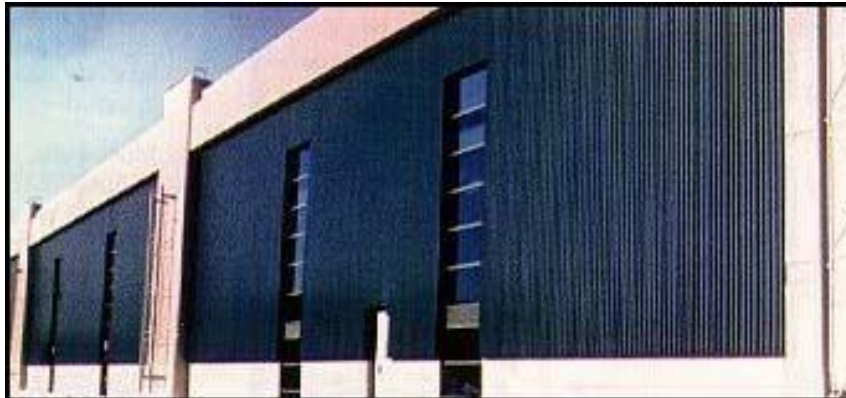
Bombardier's 10,000 m 2 (100,000 ft 2 ) SOLARWALL® is the world's largest solar air heating system
